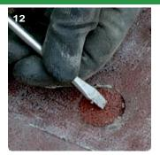
" Apply a small amount of the remaining anchor resin to the bolt heads of the shallow holes (thin covers) and the side wall of the thicker covers for the deeper holes. Fit the screw covers using a flat screwdriver to guide in. Tap in flush with a lump hammer and wipe off any residue.
