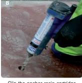
» Clip the anchor resin cartridge to the cage gun, cut off the end, attach the nozzle and squeeze the trigger to pre-mix the two components in the nozzle until a uniform mix exudes. Use the spent Roadfix container.
