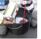
Using a second person, slowly add the liquid from the metal tin (part A), pouring over 20 seconds whilst continuing to mix.
