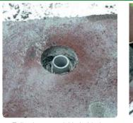
» Following on quickly behind, Insert the plugs into each hole and tap down until they are through and past the metal base bracket. Note: Forcing the coach screw and plug through together will only expand and damage it, preventing full penetration.
