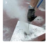
» Blow out the holes using compressed air to clear out any Roadfix residue/dust left from the drilling. Note: Wear eye protection as Roadfix adhesive can be forced up the holes with the dust.
