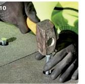
Following on quickly behind, Insert the plugs into each hole and tap down until they are through and past the metal base bracket. Note: Forcing the coach screw and plug through together will only expand and damage it, preventing full penetration.
