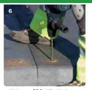
» Using an SDS drill with the 14mm drill bit provided, carefully and vertically drill out the holes to a depth of 110mm. Tip: Mark depth on bit using tape 240mm up from the drill point.
