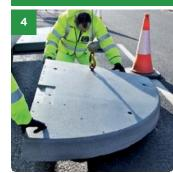
Lift the unit onto the glue bed.
